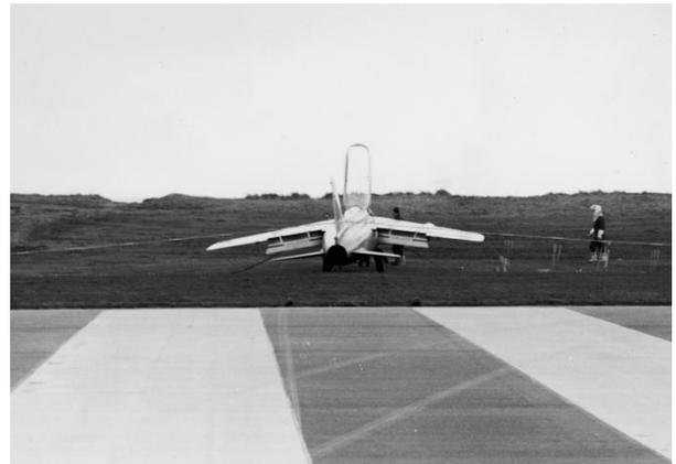
Flt Lt Baron's No 4 FTS Gnat in the barrier at RAF Valley in 1966 following brake failure on landing
